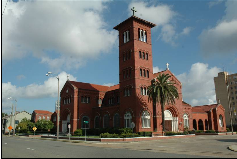
Example of a Catholic church with a Latin cross plan and bell tower.
