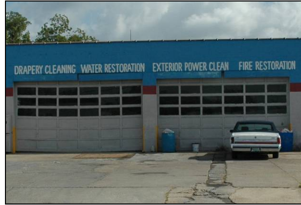
The overhead doors are character-defining features of this service-bay business.
