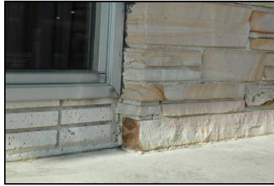
Note the juxtaposition of materials in this exterior wall.
