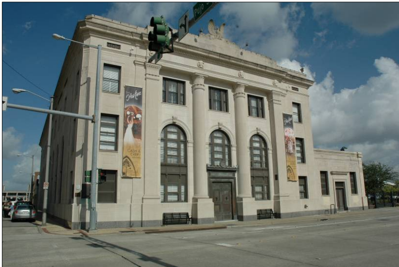
This is a Classical Revival Style commercial building with a temple front form.
