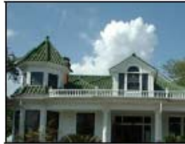
The green tile roof, cornice, balustrade, and varied roof dormers are character-defining elements of the Queen Anne Style.
