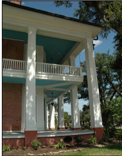
Wraparound porches and side porches that were designed to be open to the air should remain open, without screens or glass enclosures. Note the use of "Lake Charles columns" which are paneled, square, and slightly tapered.
