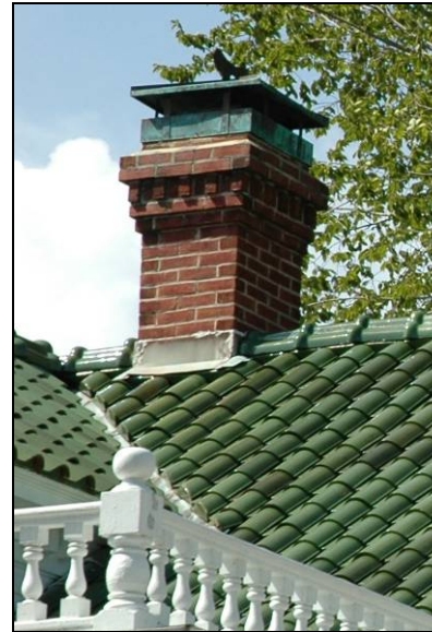
The corbelling and metal flue are character-defining features of this chimney.
