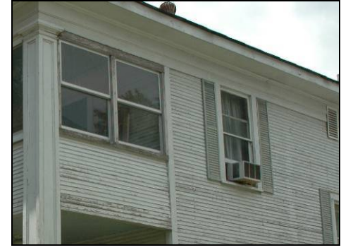
Original windows are maintained despite the installation of new HVAC units.
