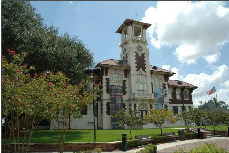
The Old Lake Charles City Hall is a central block with wings in the Italianate Style.
