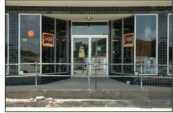
The display windows in this storefront project beyond the door, designed to call attention to the display within.
