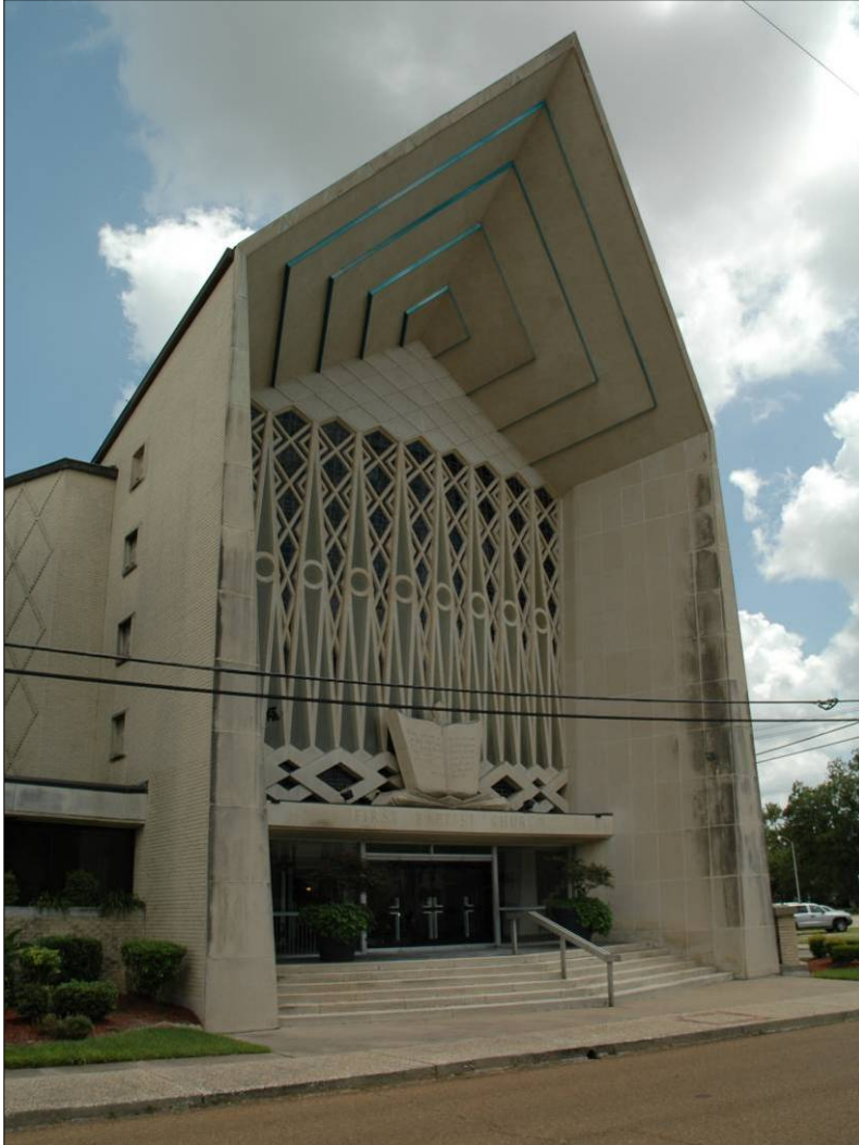
A Contemporary Style church. Note the cantilevered canopy over the entry and the angled end walls.
