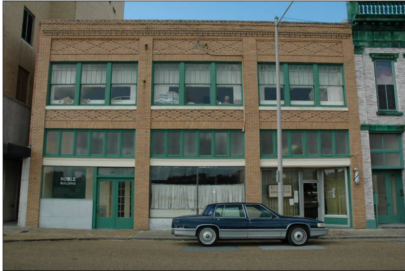
Example of a Prairie Style two-part commercial block. Note geometric detailing and storefronts.
