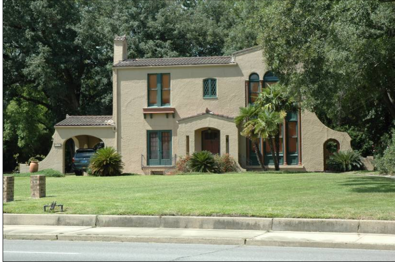
Example of a Spanish Eclectic central passage plan house. Note stucco walls with curved end walls and clay tile roof.
