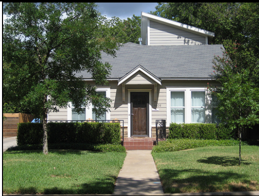
Although the scale of the addition is small, the roof form does not reflect the character of the original building. Because the form of the original building is so simple, the addition visually competes with the original building.
