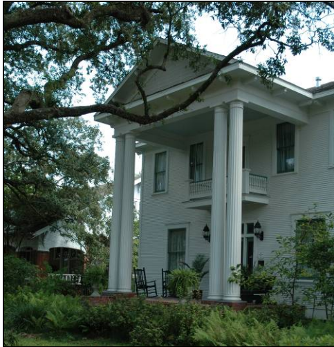
On this porch, the paired columns, cornice, and pedimented roof form are character-defining features of the Classical Revival Style and should be preserved.
