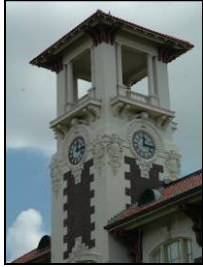
The bell and clock tower are character-defining features of this building in the Italianate Style.
