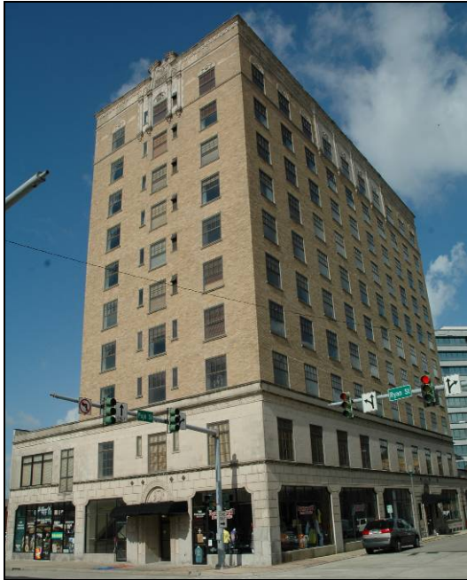
Example of a Renaissance Revival Style three-part commercial block.
