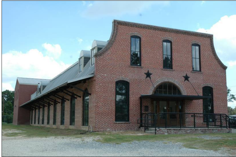
Example of a French Eclectic warehouse building. Note mansard roof behind parapet façade.
