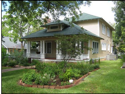
The addition is set back from the front façade and does not destroy or detract from character-defining features of the original building. The roof form from the original building is reflected in the roof form of the addition.
