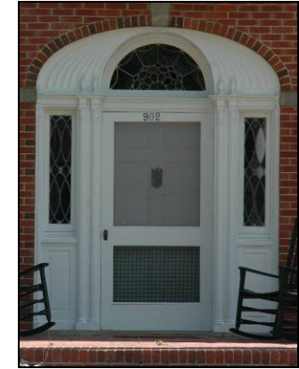
Note the segmental arched surround framing the door with sidelights and fanlight.
