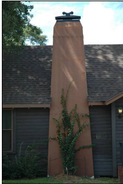
Note the tapered form of the chimney on this Craftsman Style house.
