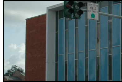
Use of multiple materials is a character-defining feature of some buildings. Note the glass and ceramic spandrel curtain wall.
