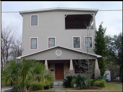
The addition is set forward flush with the front façade. The three-story scale overwhelms the original building. The roof form and fenestration pattern do not reflect the character of the original building.
