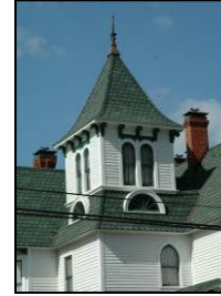
Note pyramidal roof, brackets, and eyebrow dormers at this tower on a home with Queen Anne elements.
