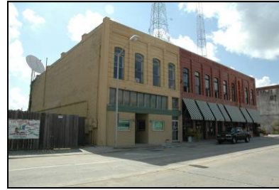
A canopy that runs horizontally between the transom above and the storefront below (left) is appropriate. Canopies and awnings should avoid covering windows or transoms.
