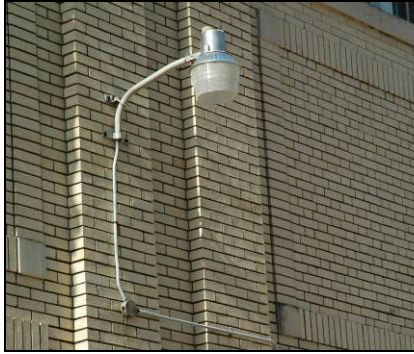
Here, mechanical features are mounted on a side façade.
