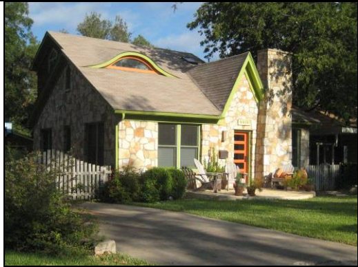
To accommodate the addition, the roof has been elevated slightly and a dormer window has been added, but the original roof form is maintained. The scale of the original building is maintained.
