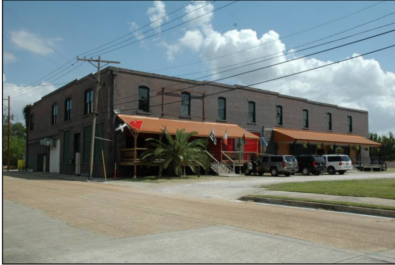
Example of a warehouse. Note loading bays.
