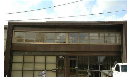
The casement windows at the storefront and ribbon windows in the transom complement the façade of this enframed wall Modern building.
