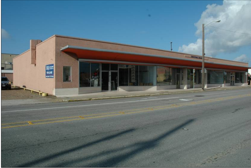
Example of a Moderne one-part commercial block. Note cantilevered canopy.
