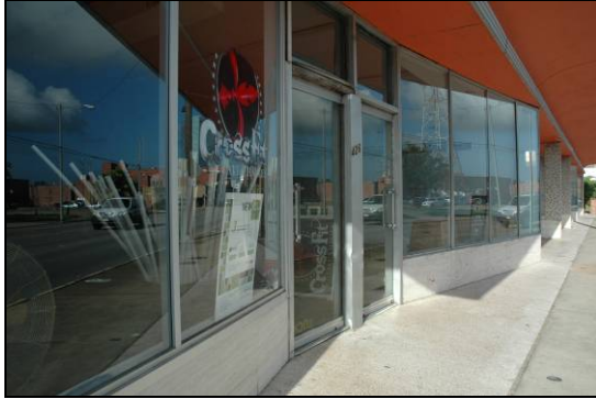
Note the proportion of glass to metal in this storefront's doors and windows, as well as the terrazzo flooring at the entry.
