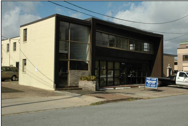
Example of a Modern enframed window wall building. Note storefront and projecting elements framing the façade.
