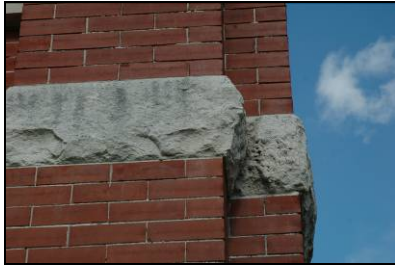
The character of an exterior wall is defined by its texture, color, and pattern. Note use of brick and stone string course.
