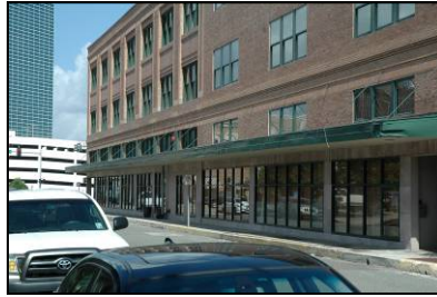
The metal canopies of these adjacent buildings are consistent in design and form and feature metal support rods. Note the canopies' subtle downward slope.
