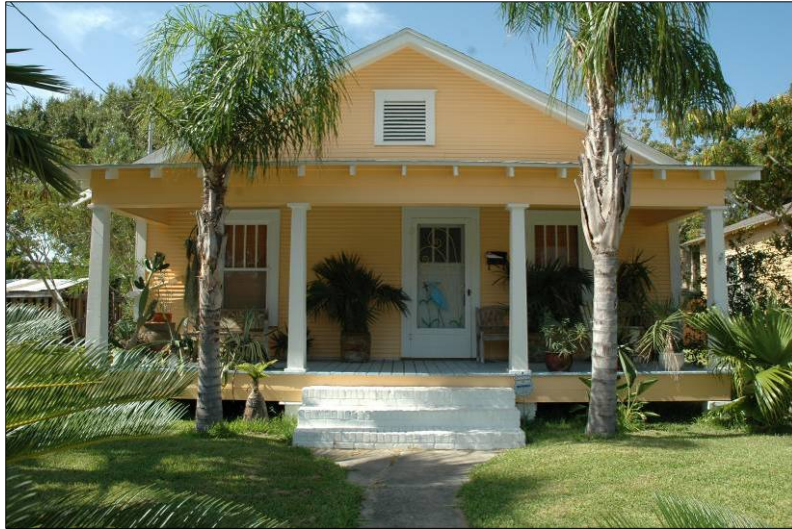
Example of a Craftsman Style bungalow. Note exposed rafter and tapered porch supports.
