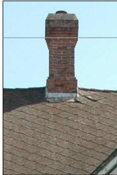
Note the height of the chimney.
