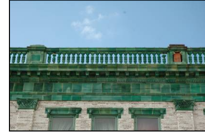
The terracotta roof parapet with balustrade and cornice is an important feature of this Italianate commercial building.
