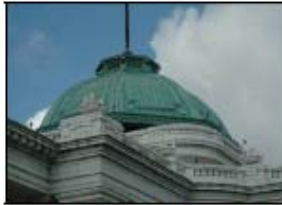
On this Classical Revival government building, the molded cornice, roof balustrades, and dome are important character-defining features.
