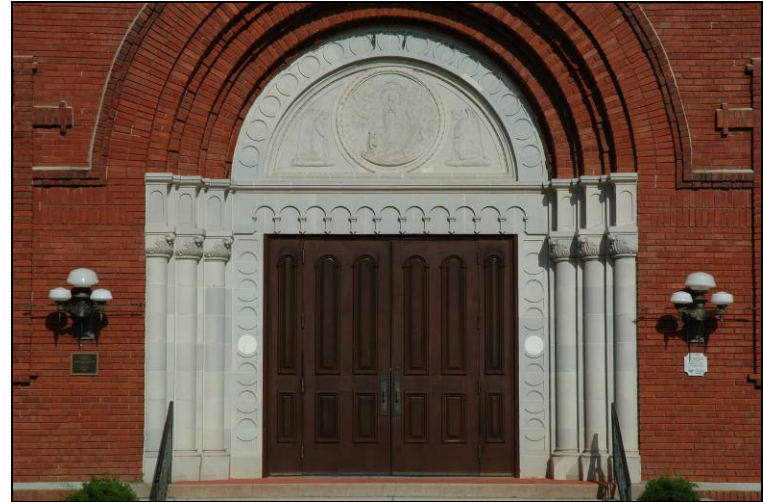
The graduated recessing of the arches and columns form an entry porch at this Romanesque Revival Style church.
