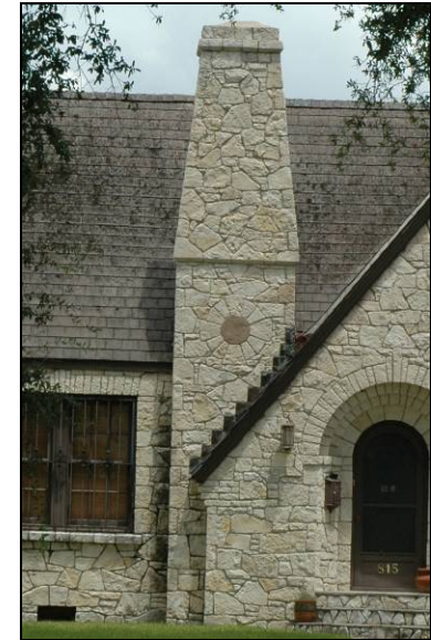
Note the relationship between the width of the chimney and the width of the front façade.
