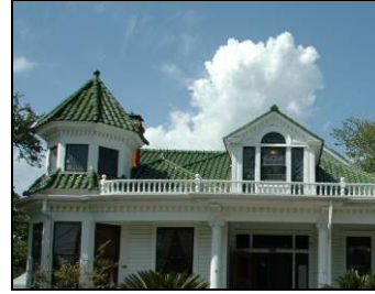
The green tile roof, cornice, balustrade, and varied roof dormers are character-defining elements of the Queen Anne Style.
