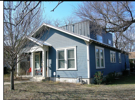
The addition is set forward almost flush with the front façade of the original building. The flat roof is not compatible with the character of the original building. Modern or Contemporary design may be appropriate for an addition, provided that it is not visible from the street.
