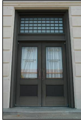
Note the proportions of the doorway and of the glazing to the wood.
