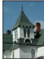
Note pyramidal roof, brackets, and eyebrow dormers at this tower on a home with Queen Anne elements.
