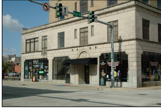
The storefront in this three-part vertical block is emphasized by larger windows, a recessed entry, different wall materials, and ornamentation.
