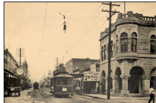
Views of Ryan Street in 1905 (Louisiana Digital Library): Top: looking south from Division Street Center: looking north from Pujo Street Bottom: looking south from the corner of Broad Street
