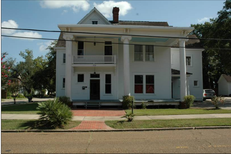
Example of a foursquare Classical Revival house with a rear addition. Note the porch with monumental columns.
